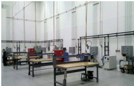
SMC US Repair Facility
